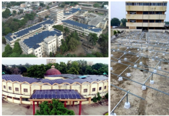
Title : 750 kWp Grid Connected Roof Top Solar Power Plant at Dr. PDDMMC Location : Amravati Year of Installation: 2019
