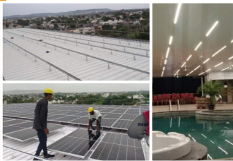
Title : 150 kWp Grid Connected Roof Top Metal Profile Shed Solar Power Plant at Rangoli Hotel Location : Amravati Year of Installation: 2021
