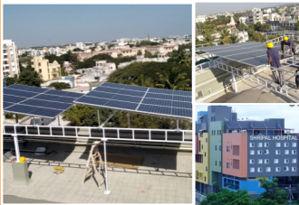
Title : 140kWp Grid Connected Super Structure Type Elevated SPVPP at Shripal Hospital Location : Baramati Year of Installation: 2022
