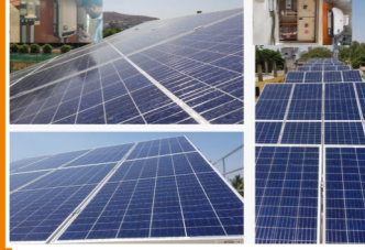
Title : 25 kWp Grid Connected Roof Top Solar Power Plant at Vidyanchal School Location : Pune Year of Installation: 2021
