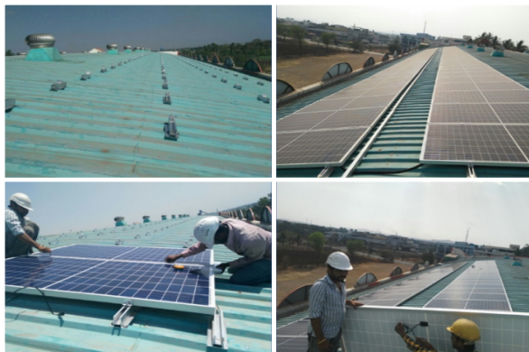
Title : 30 kWp Grid connected Metal Profile Roof Top Shed Solar Photovoltaic Power Plant at SYM Hall Location : Islampur, Sangli Year of Installation: 2017
