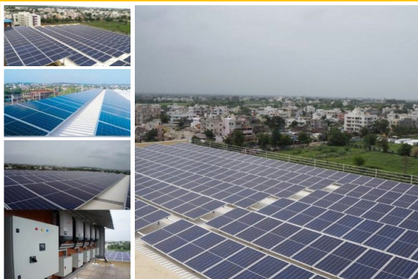
Title : 125 kWp Grid Connected Metal Profile Roof Top Shed Solar Photovoltaic Power Plant Location : Amravati Year of Installation: 2017
