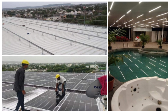
Title : 150 kWp Grid Connected Roof Top Metal Profile Shed Solar Photovoltaic Power Plant at Rangoli Hotel Location : Amravati Year of Installation: 2021
