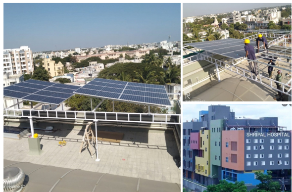
Title : 140kWp Grid Connected Super Structure Type Elevated SPVPP at Shripal Hospital Location : Baramati Year of Installation: 2022
